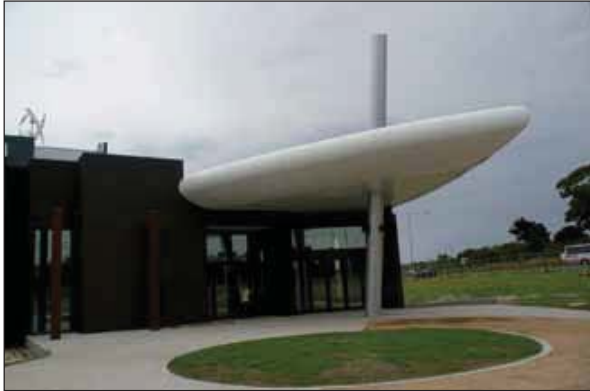
Environmental protection and sustainability are valued highly on the Surf Coast. The efficient building system technology with KNX meets this requirement
