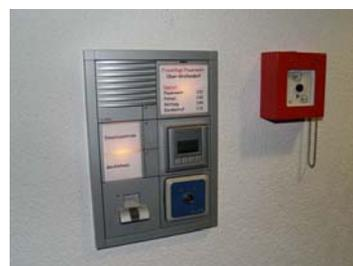
**Figure 2. Thanks to the networking of the various trades, the doors are opened and the lights switched on via fingerprint access control. Source: HTL St Pölten**
