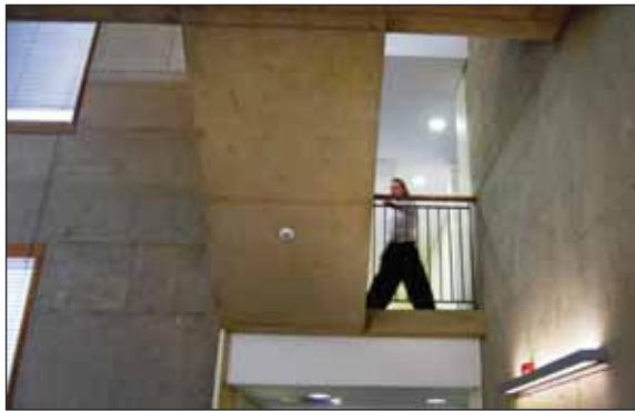
Picture 2. Energy Efficiency 2: Lots of daylight and presence sensors for the lighting system.
