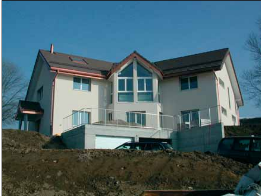
Figure 1. Single family home in Puidoux with high energy efficiency due to KNX
