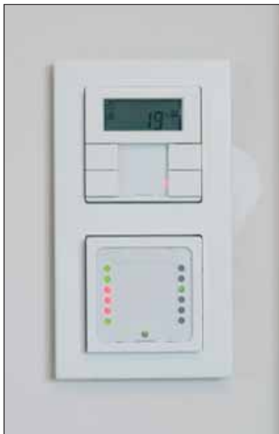
Figure 2. KNX multi functional operating panel in the rooms: temperature sensor, display, button for lights and shading, LED display
